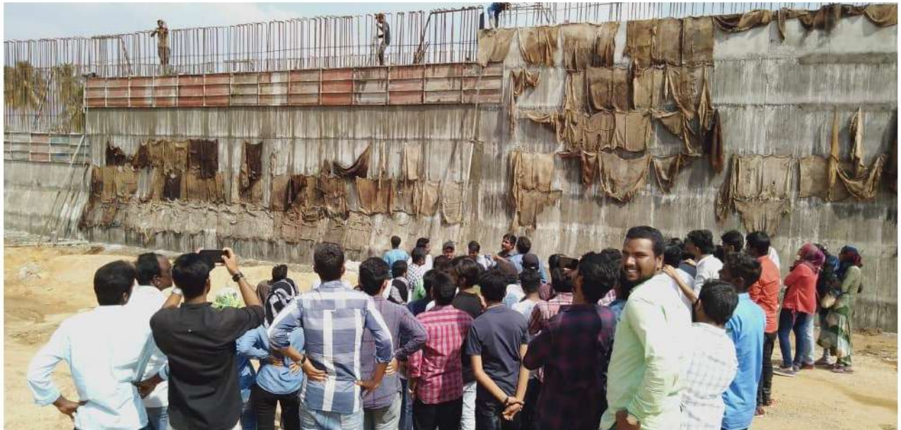
Upper Bhadra Project tunnel wall
