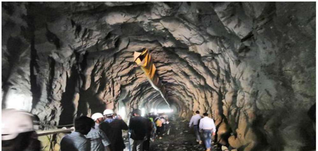
Upper Bhadra Project tunnel.
