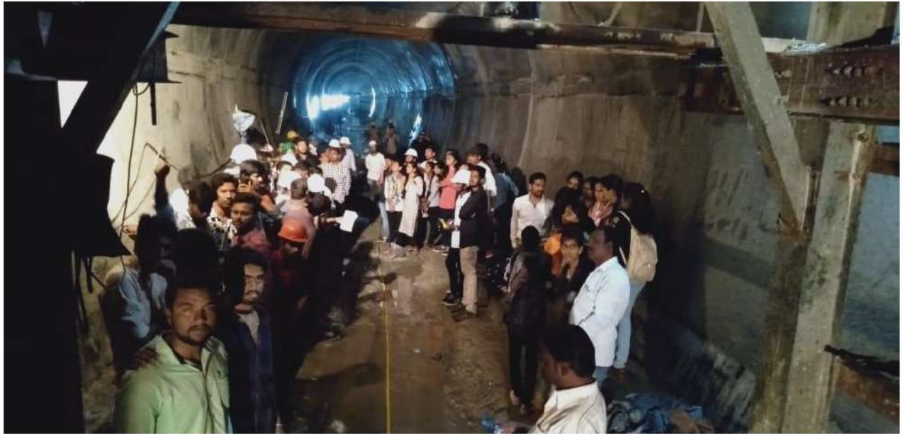
Upper Bhadra Project tunnel.
