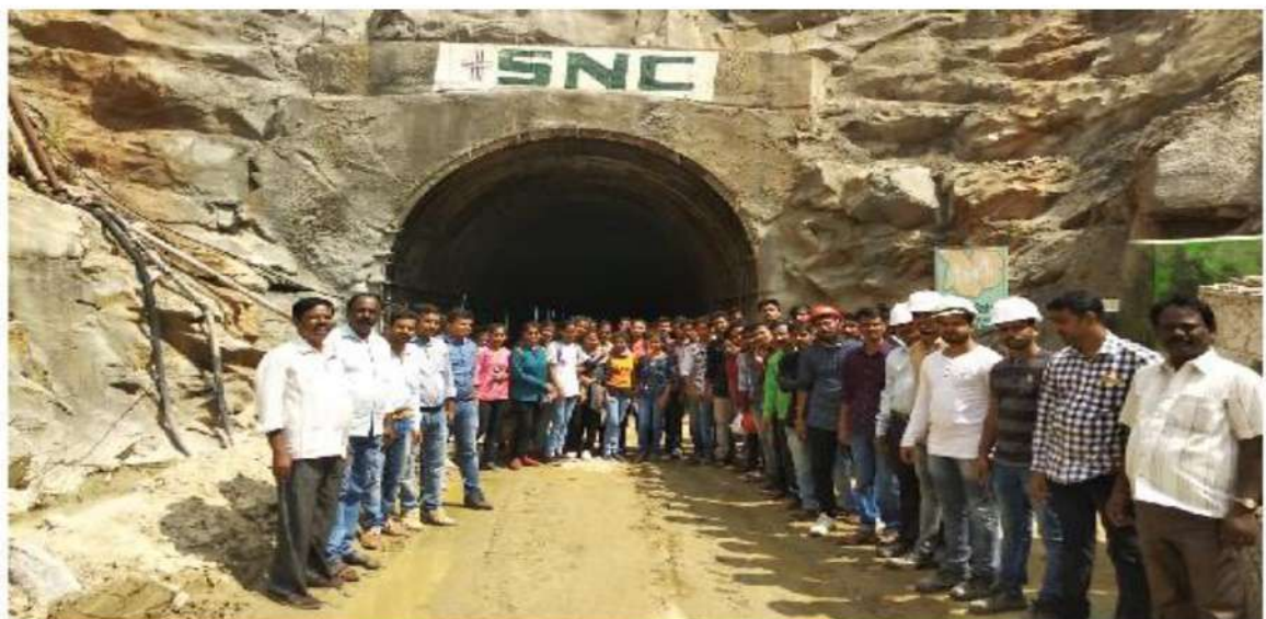
Upper Bhadra Project tunnel.
