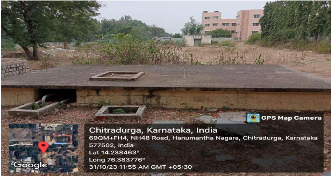
Photo 11: Sump for Collection water tank
