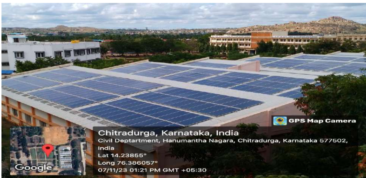
Photo 2: Solar system on Non-IT Block
