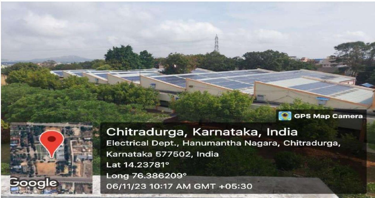
Photo 1: Solar system on Non-IT Block
